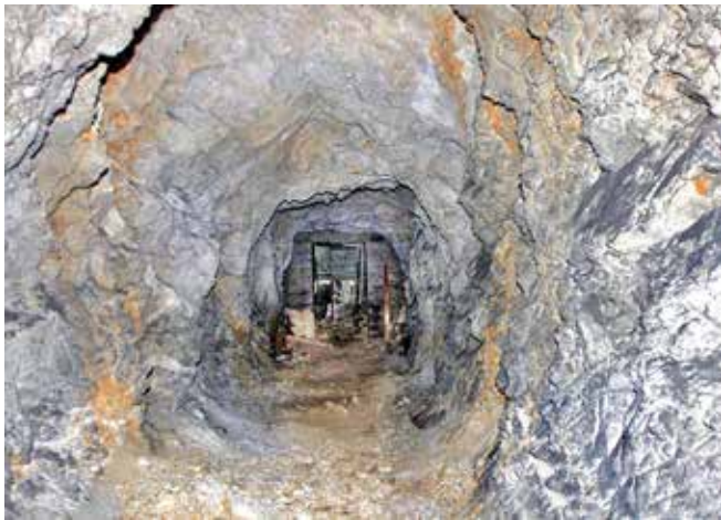
Looking east towards the entrance from the first junction in Bunker 1. Photo Žiga Ribič
